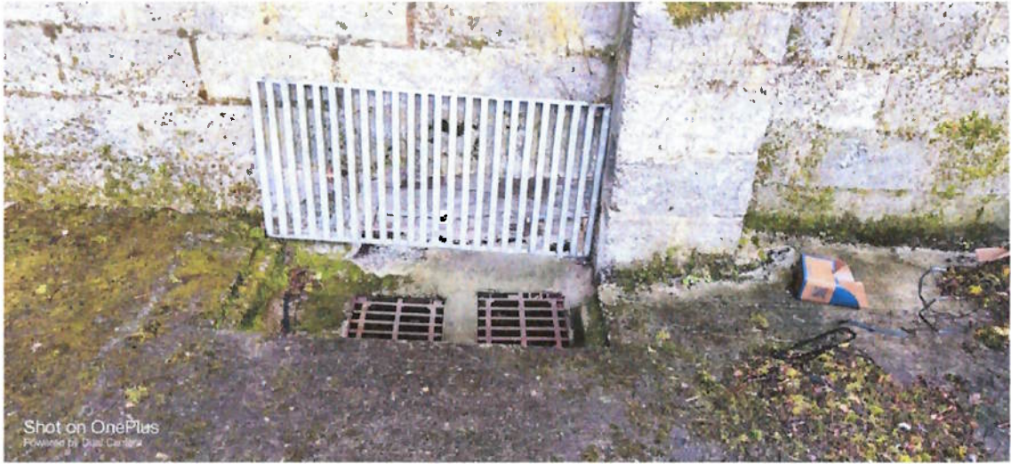
Drain to rear of current wall
