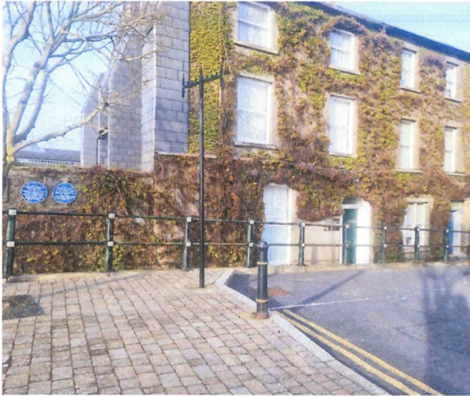
Georgian Terrace with Original Railings
