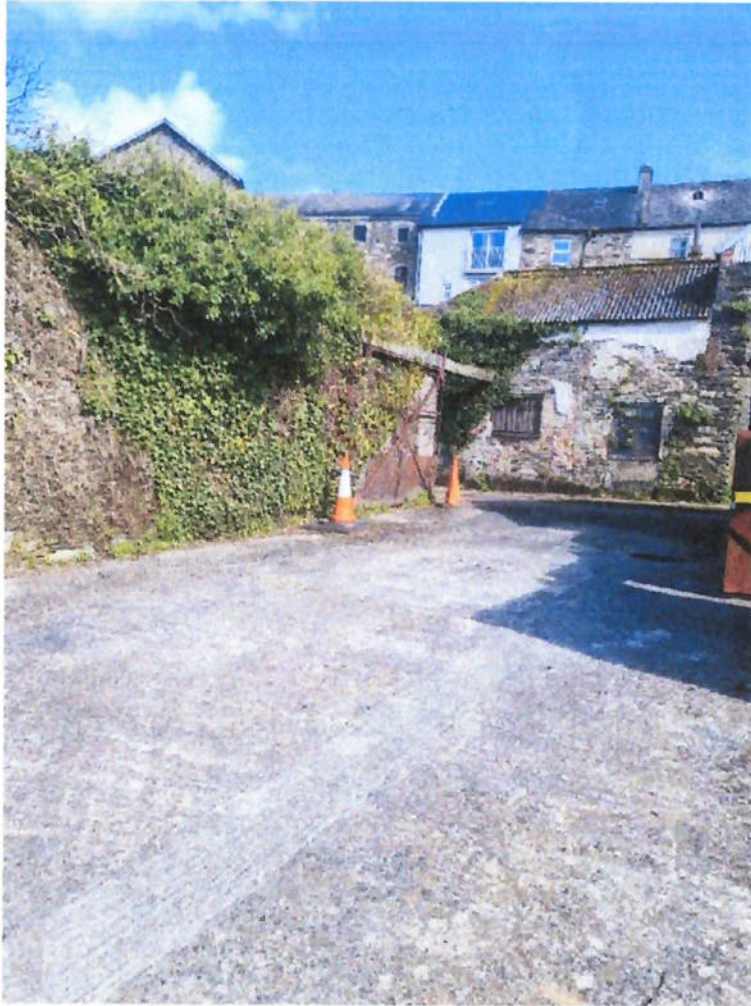
Private Property to rear of Nos. 1 & 2 Bridge Street
