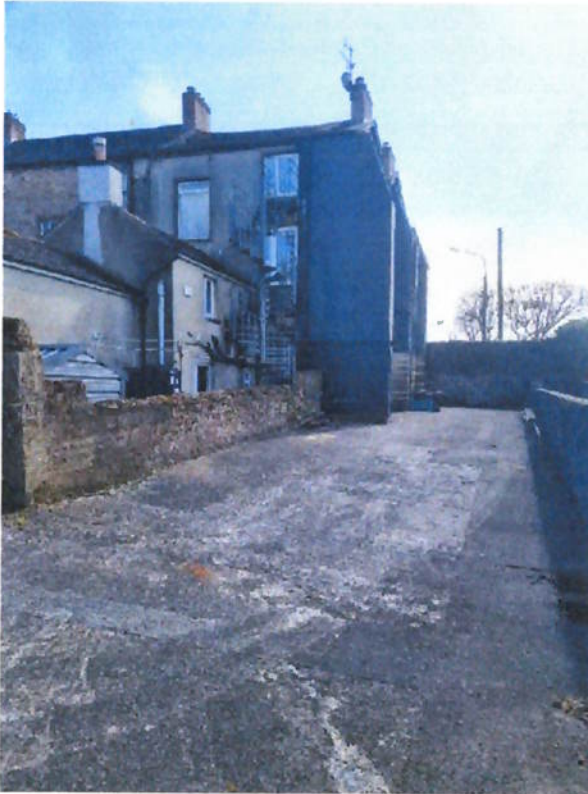
Rear View of No.2 Bridge St. – Rogers Dental
