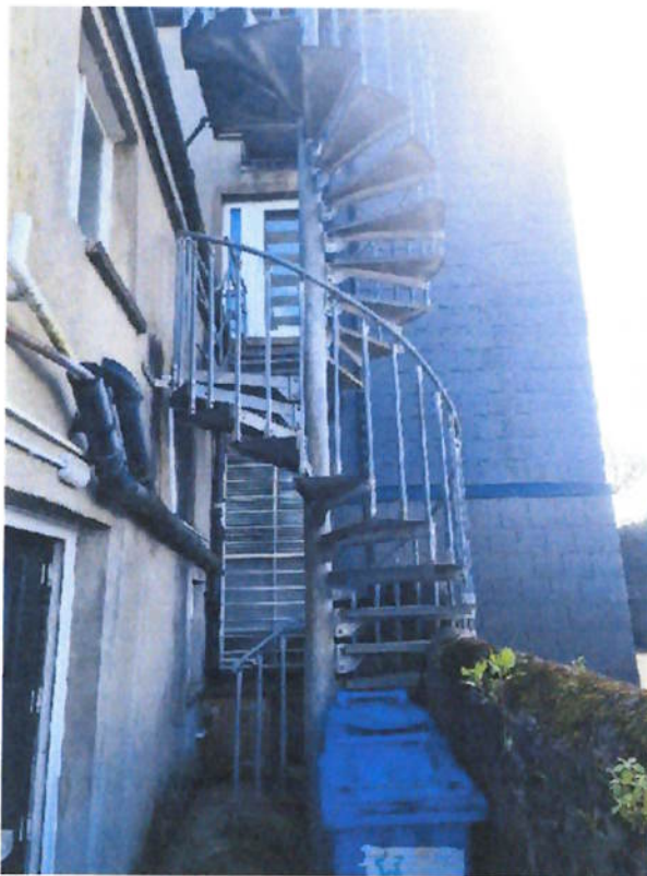
Fire Escape to rear of Property
